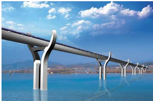
Geumga Extradosed Bridge
